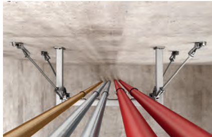
Bracing of frame construction with threaded rods
