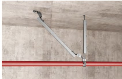
Bracing of pipeline with channel profiles
