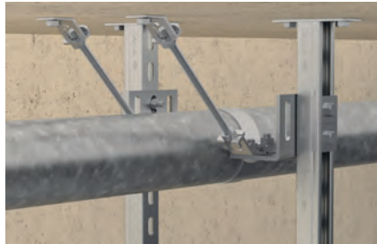
Bracing for fixpoint
