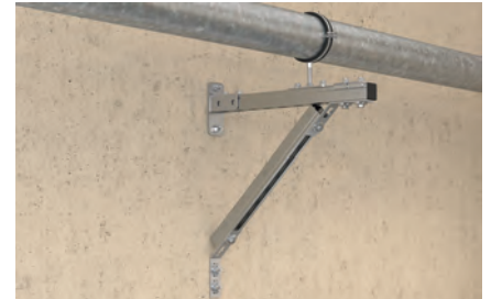
Upright pipe on cantilever arm
