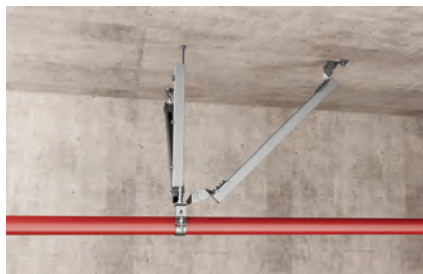
Pipe installation with seismic pipe clamp
