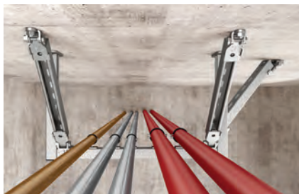
Bracing of frame construction with channel profiles
