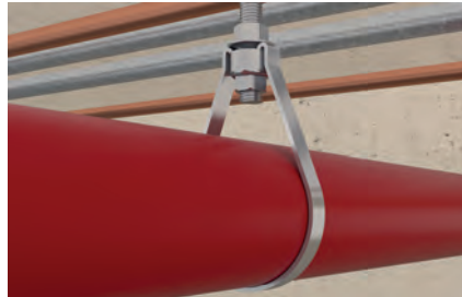
Sprinkler pipe installation
