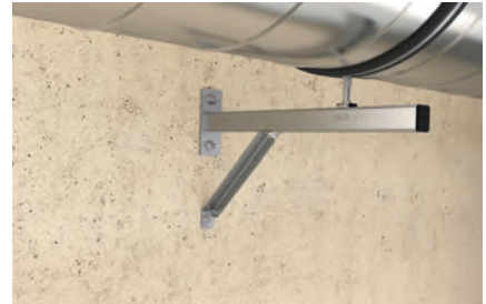
Ventilating pipe fixing at the wall
