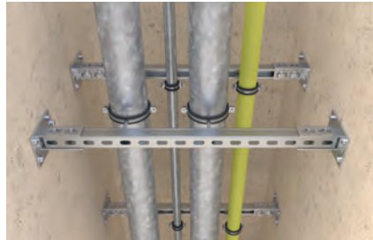
Pipe installation in escape route
