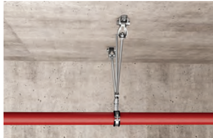
Bracing of pipeline with threaded rods
