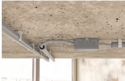
Fixing plastic insulating conduits
