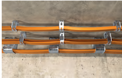
Cable fixing to the ceiling
