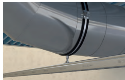
Support systems for ventilation
