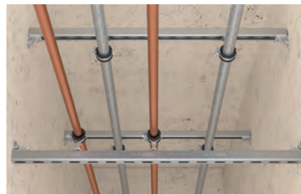
Pipe fixing in a corridor
