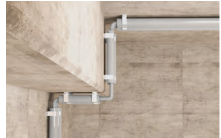
Fixing plastic insulating conduits
