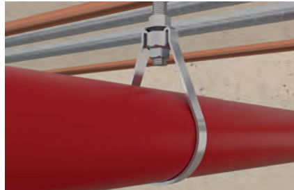
Sprinkler pipe installation
