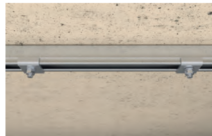
Channel installation at wall
