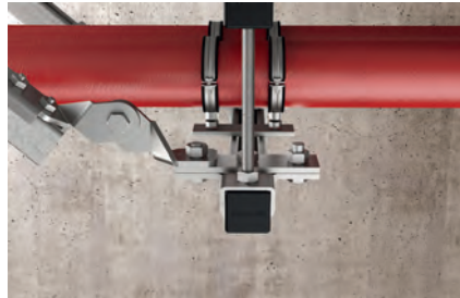
Bracing of channel construction
