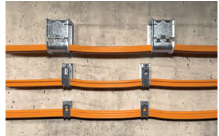
Cable fixing to the wall
