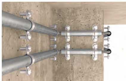
Fixing steel armoured conduits
